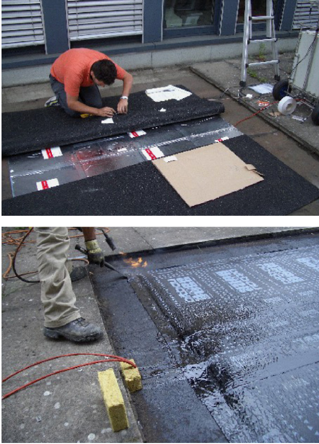
Fig. 4. Pictures from the installation process of the two VIP test areas.
